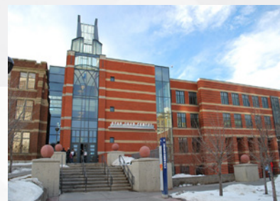
STAN GRAD CENTRE SOUTHERN ALBERTA INSTITUTE OF TECHNOLOGY (SAIT)
