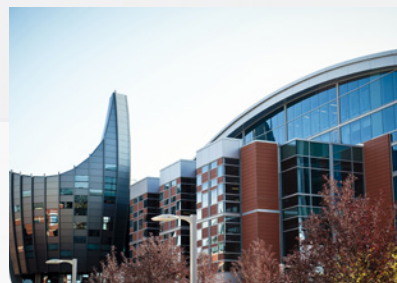
JOHNSON - COBBE ENERGY CENTRE SOUTHERN ALBERTA INSTITUTE OF TECHNOLOGY (SAIT)
